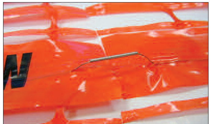
Connection of the mesh using the crimps. If the mesh wire is not installed correctly then the signal may not pass from join to join.
