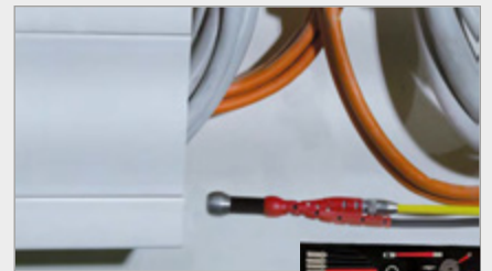
Shafts and underfloor ducting
