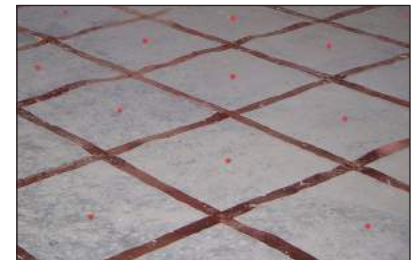
Pedestal locations marked by the dot
