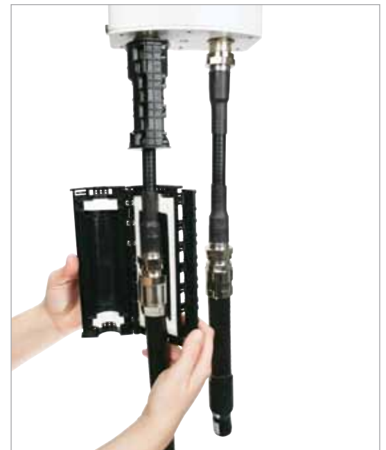
Installation of the 3M™ One Step Closure for Wireless OSCW-F-7/8
