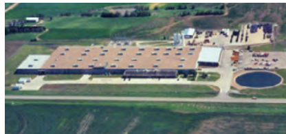
Hoisington Communications Plant | Hoisington, KS
